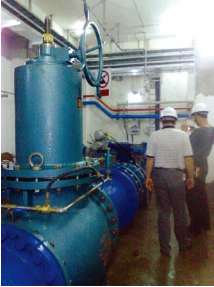
ZJY46H减压阀在构皮滩电站的应用 The application of ZJY46H pressure reducing valves in Goupitan Power Station
